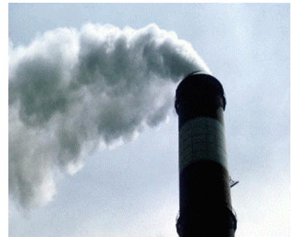
Chimney stack emissions
